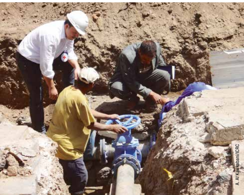
An ICRC engineer and local water board member connect the main public water pipeline to a district in the Yemeni city of Sana’a. December 2016.
