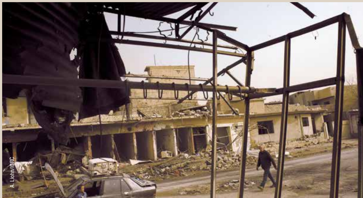
Damaged residential area in eastern Mosul. February 2017.
