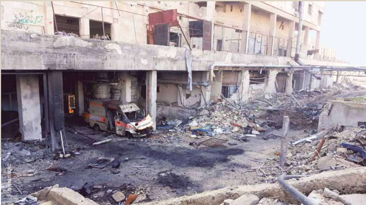
Scene of destruction after Aleppo National Hospital came under fire. January 2017.
